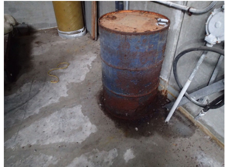
Leaking of an unknown liquid from 55-gallon drum located on the back wall of the ground floor.
